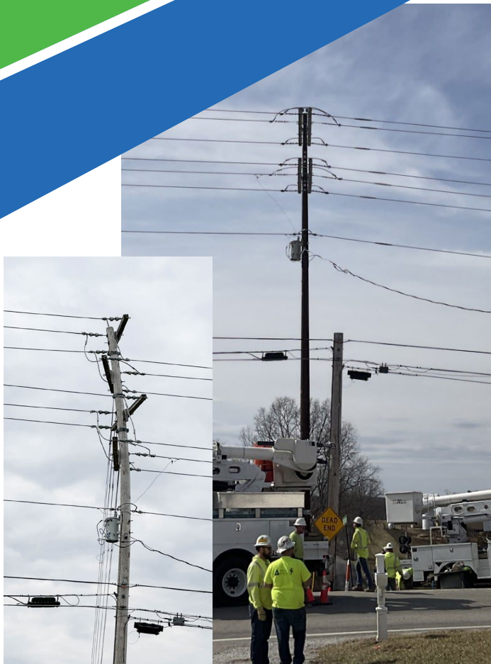
Pole Replacement Before & After
